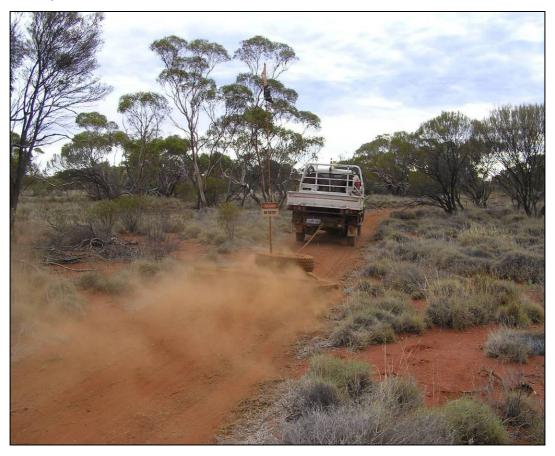
Plate 2-1 "Clearing" Road Route with Tyre Grader
