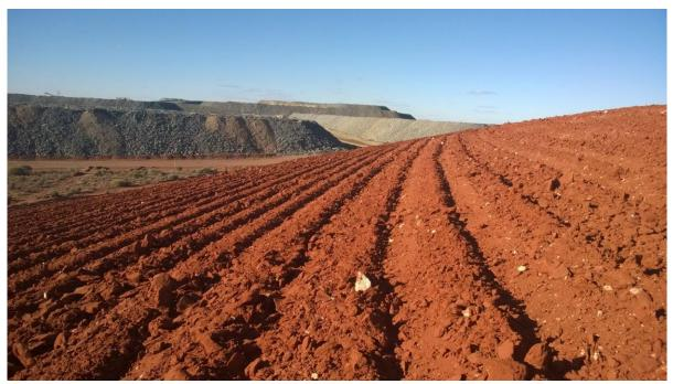
Figure 1: Contour ripping trial across the entire LWE batter.
