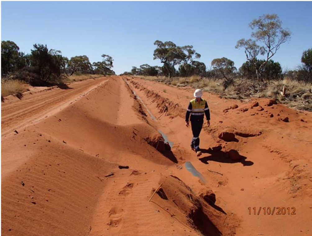
Plate 5: Fauna trench inspections – Process Water Supply Area pipeline
