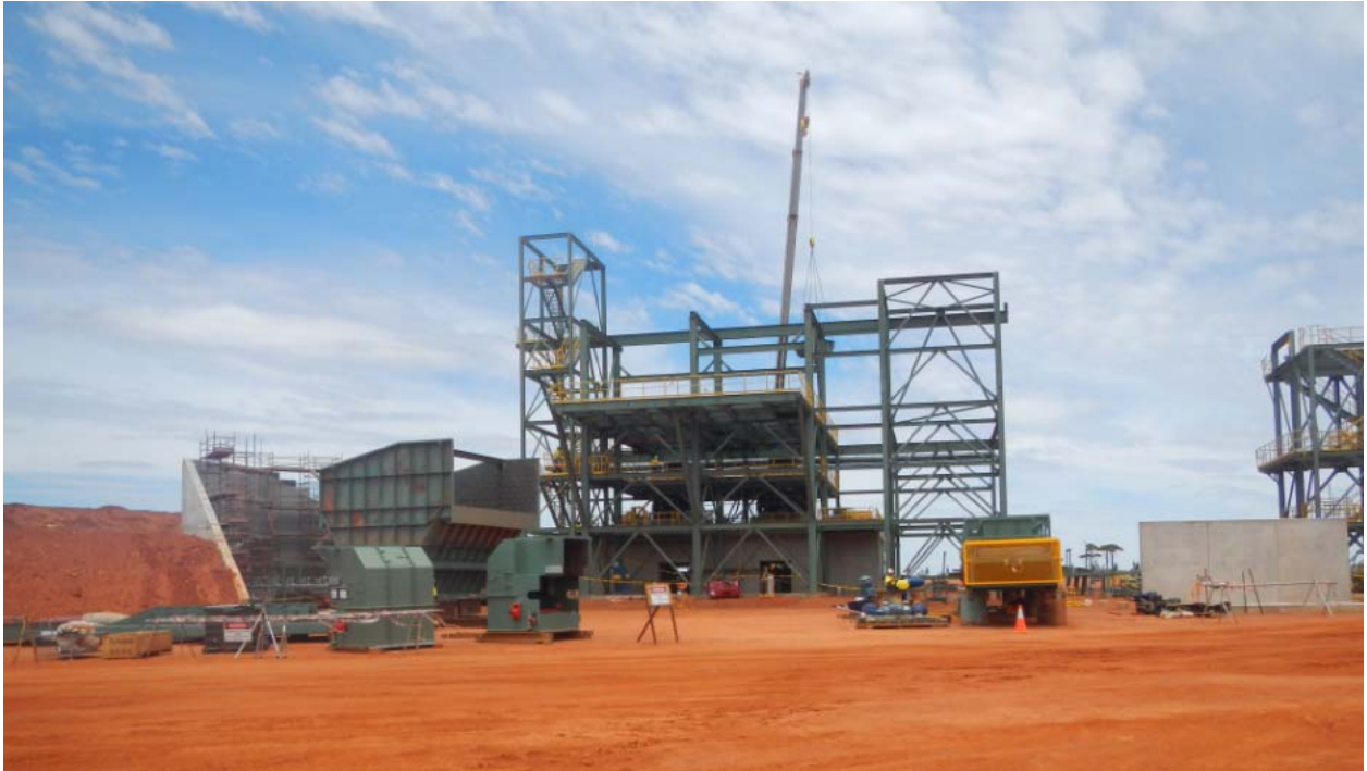
Plate 3: Processing Plant Construction - Crushing circuit
