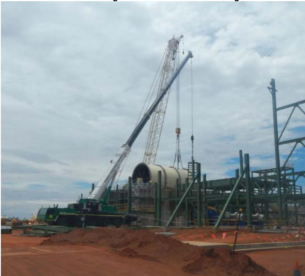
Plate 4: Processing Plant Construction – Ball Mill
